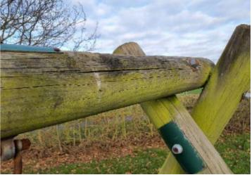
**Finding:** The timber has a number of splits/shakes or air **Action:** Monitor to ensure the splits do not cross through cracks and this may affect the stability or allow water ingress fixing points of the structure and/or cause any instability which will accelerate the rotting process
