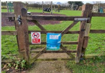
**Finding:** There are openings that are less than 12mm that could trap or crush fingers
