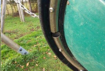
**Finding:** There is / are post or end caps missing / damaged **Action:** Replace missing / damaged post or end caps on the item
