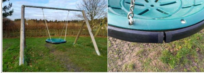
Finding: The joint collar is missing Action: Replace
