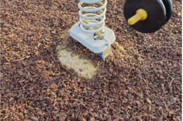
**Finding:** The depth of the loose fill surfacing is lower than the recommended depth specified in BS EN 1176 exposing the concrete foundations; the free height of fall of the equipment is less than 2.0m and a minimum of 300mm depth should be provided (including an extra 100mm to allow for compaction and displacement as per BS EN 1176 Part 1 - Table 4)
