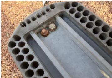
Finding: The fixings have corroded excessively
