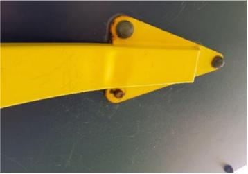
Action: Replace all corroded fixings
