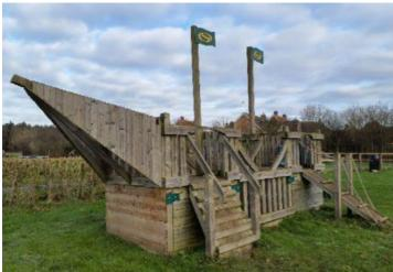
**Finding:** The access ramp height is greater than 600mm and the angle of ascent is less than 38 degrees. Barriers or guardrails are required to comply with the requirements BS EN 1176
