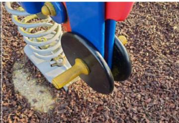
Finding: The end of handgrips and/or footrests have a cross Action: Monitor - No action given the risk assessment section of less than 15cm2 and fail to meet the requirements of BS EN 1176 Part 6
