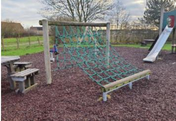
**Finding:** The table forms a hard object within the falling space of the equipment and there is also insufficient surfacing provided in contravention of BS EN 1176 Part 1
