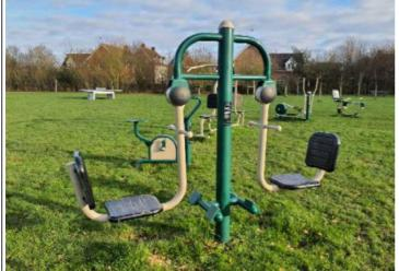
**Finding:** There is no instruction label provided; an instruction label should be provided with each item of equipment in accordance with the requirements of BS EN 16630
