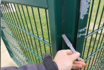
**Finding:** BS EN 15312 states that gaps whose dimensions Action: Ensure crushing hazards are removed change during use shall have a minimum dimension of 18mm
