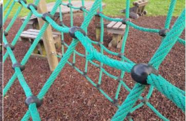
**Finding:** The ropes/nets are worn/damaged in places
