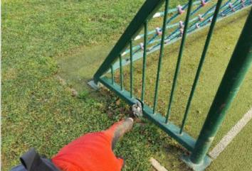
**Finding:** The goals are not securely fixed to the surface ( only by the padlock brackets which appear to be loose in the foundations)
