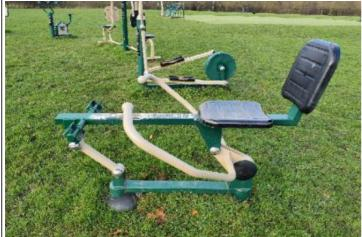
**Finding:** The signage is faded; an instruction label should be provided with each item of equipment in accordance with the requirements of BS EN 16630
