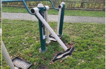
**Finding:** The swinging movement of the item exceeds the maximum 55 degrees from the vertical required by BS EN 16630
