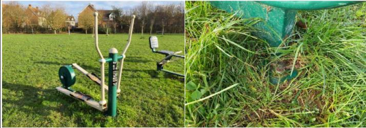
Finding: There is/are bolt cap covers missing or damaged Action: Replace missing or damaged bolt cap covers on the item
