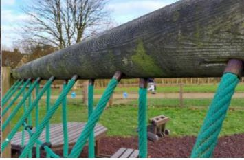
**Finding:** The fixings are corroding
