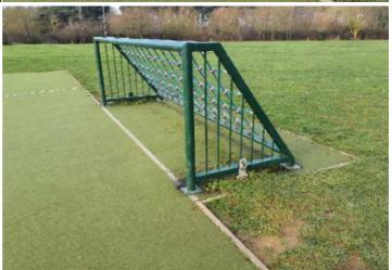
**Finding:** The design of the equipment may encourage climbs onto the goal, and the concrete edgings form an hard the design to comply with the requirements of BS EN 15312 object in the impact area in contravention of BS EN 15312
