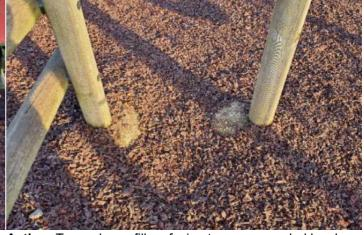
**Finding:** The depth of the loose fill surfacing is lower than the recommended depth specified in BS EN 1176 exposing the concrete foundations; the free height of fall of the equipment is less than 2.0m and a minimum of 300mm depth should be provided (including an extra 100mm to allow for compaction and displacement as per BS EN 1176 Part 1 - Table 4)
