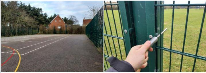
**Finding:** There is/are finger entrapments in the panels and **Action:** Monitor - No action given the risk assessment the item fails to meet the requirements of BS EN 15312
