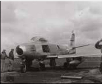
F-86A Sabre fighter of the 91st Fighter Interceptor Squadron at RAF Bentwaters in 1952. The aircraft is undergoing checks to align the guns, a procedure carried out on the boresight range. Photo Louis Schutzenberger via BCWM archives
